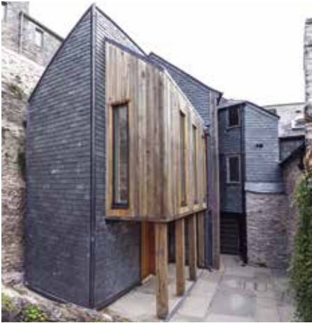
Above The new oak and Delabole slate rear extension
