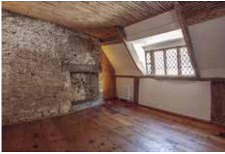
Above The top floor room following repairs
