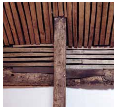
Top Rotten window cill and frame members uncovered for repair
